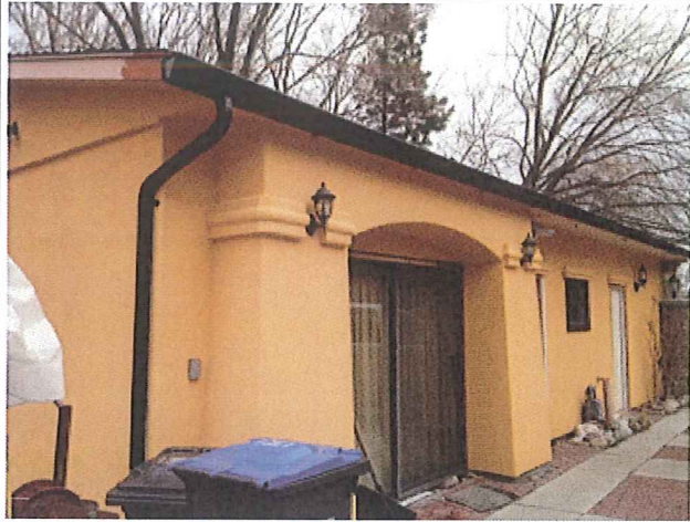
West elevation of accessory building.
