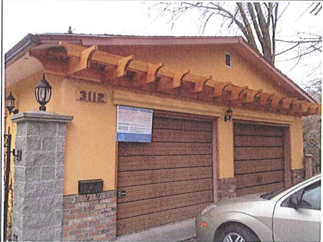
South elevation of accessory building.
